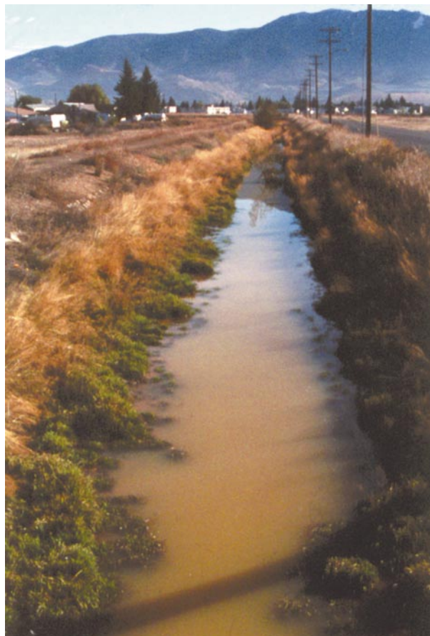
Fig. 2 Photograph of Butte's Metro Storm Drain, taken in November 1997. Note the high turbidity (despite low flow and no precipitation for several weeks), due to abundance of suspended iron oxy-hydroxide particles.
